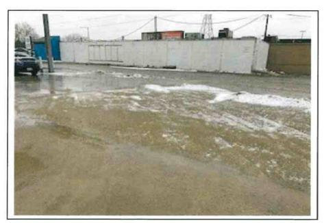
**DESCRIPTION:** View of UST excavation backfilled and capped with CA-6 rock.
