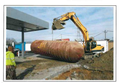
**DESCRIPTION:** View of UST removed and preparing to be cut/cleaned
